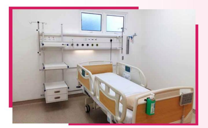
It is using double layer bed head 380mm series with 4 x horizontal rails, 2 mounted on bed head while the other 2 mounted on wall.
